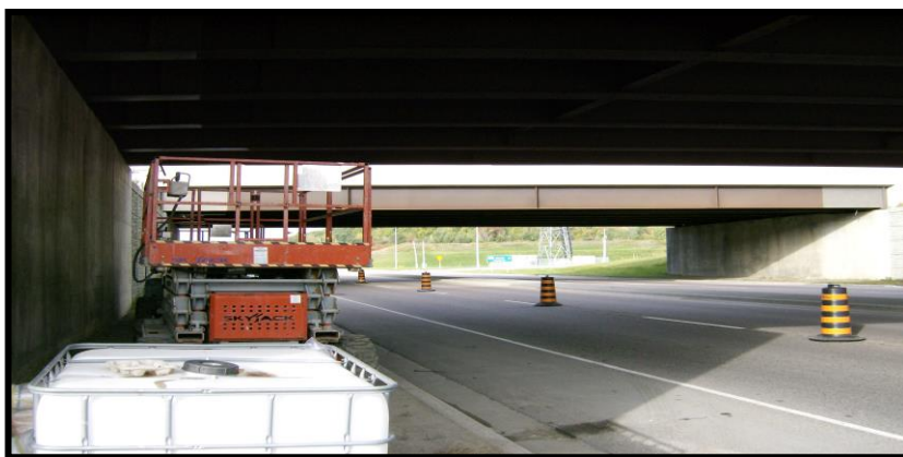
Highway underpass treated with VAPPRO 887 MAGTAN
